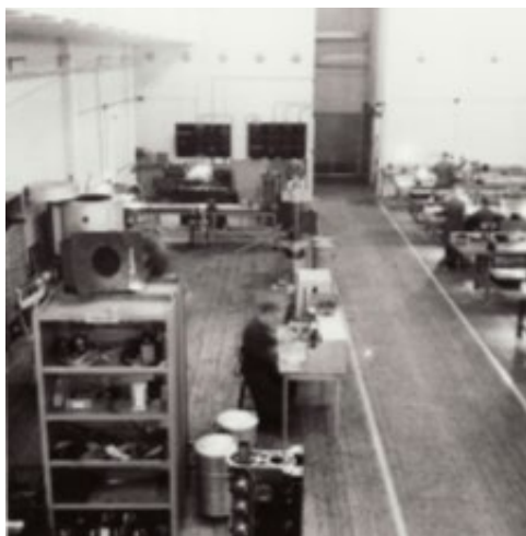
Reparationsavdelningen tunnel III 1946.
